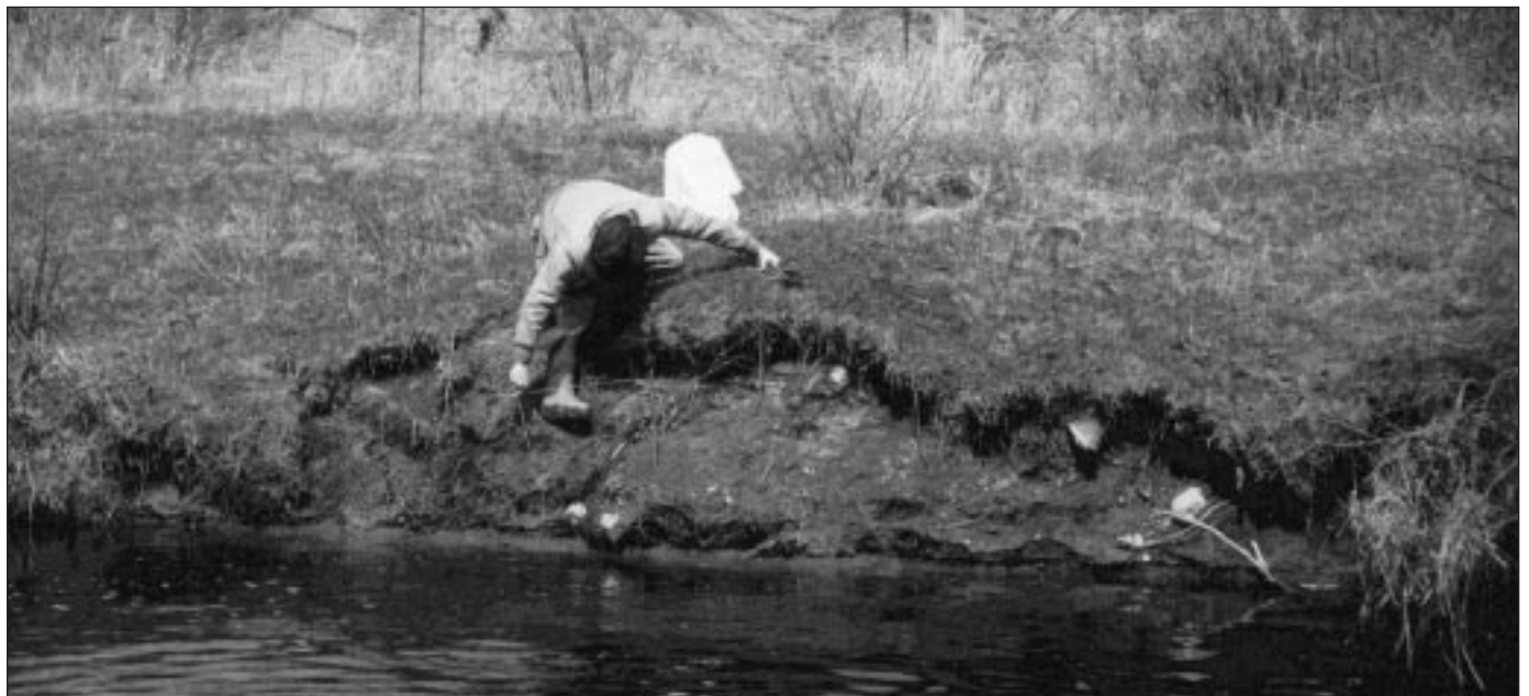
Figure 2 — Plant the lowest row of willows just below the high water mark of a stream, river or lake.
